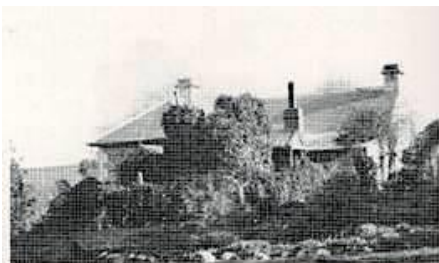
Lily Bank homestead on Cookes Hill Road. The John Thomson family built the first portion of this house in the late 1850s. Until the early twentieth century, Francis Thomson lived here. The Thomsons then sold the property to other folk.
