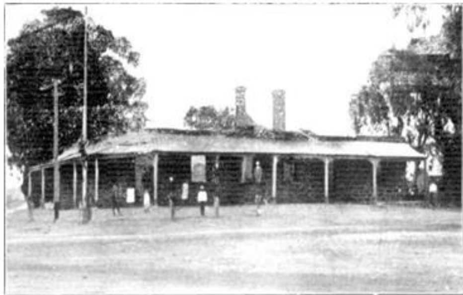
Travellers Rest Hotel showing badly damaged roof after 1914 fire
